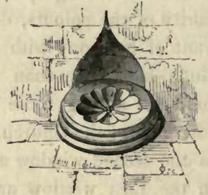
Water Drain, in Vestry.
